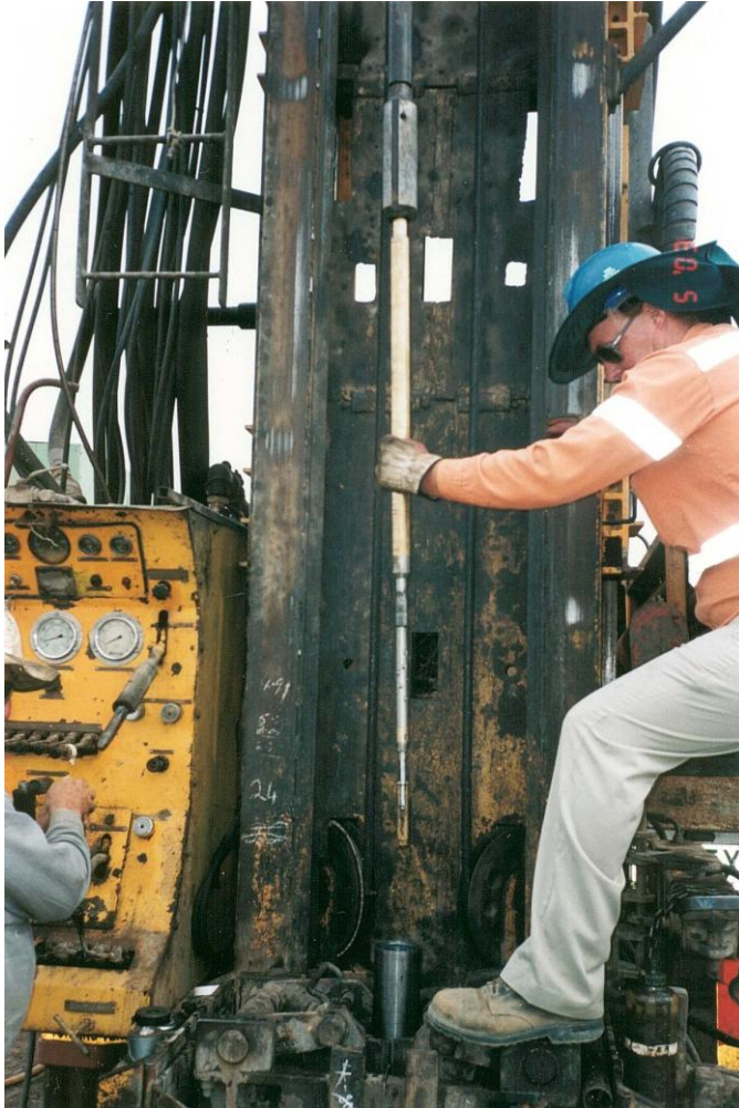
A Sibra in-situ stress measurement tool about to be lowered through an HQ drill string.
