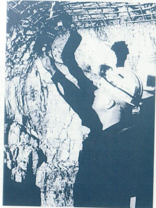
(Figure 2). Use of Methane Detector (Mentor)
