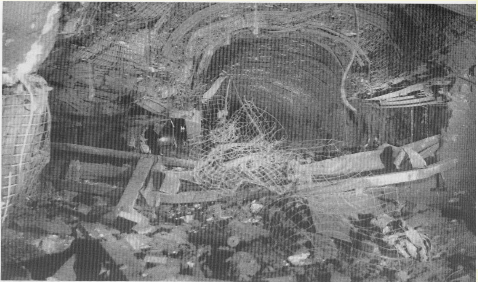
Fig. 404 Explosion damage underground - Appin Colliery
